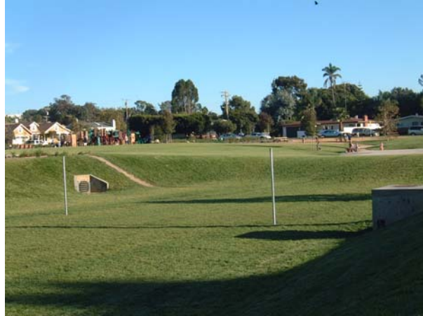
Photograph: City of Encinitas, Volleyball Court/ Detention Area
