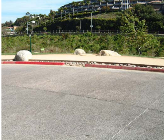
Photograph: City of Encinitas, Permeable Pavement & Rock Edge
